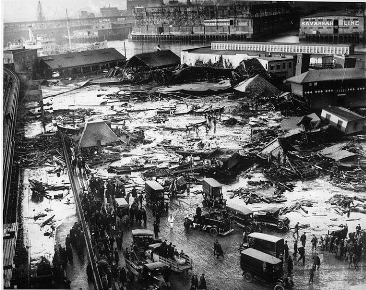
Figure 1. Aftermath of molasses tank failure
